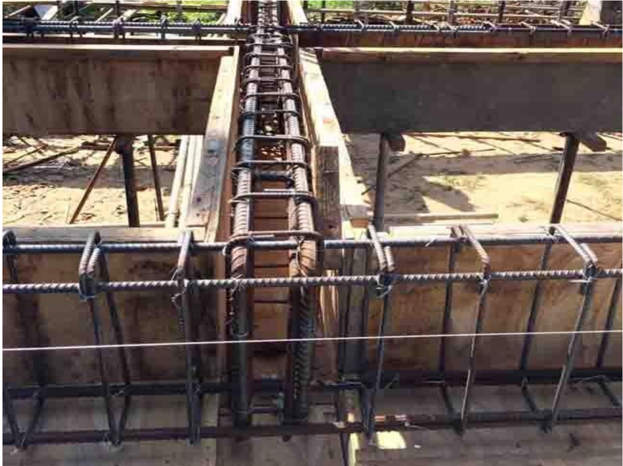
Reinforcement detailing for beam on the site
