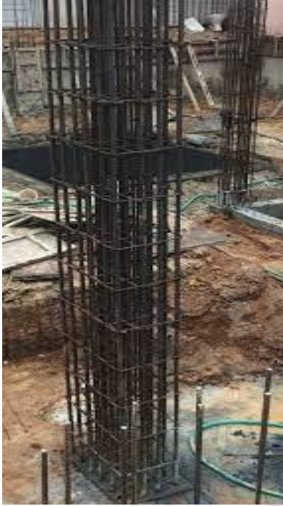
Reinforcement detailing for column in site
