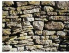
Un-coursed Rubble masonry
