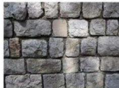
Third class coursed rubble masonry
