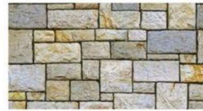
Second class coursed rubble masonry
