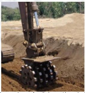
a. Compaction reduces volume of soil by rapid mechanical methods like tamping, rolling and vibration; whereas consolidation process reduces volume gradually bystatic, sustained loading.
