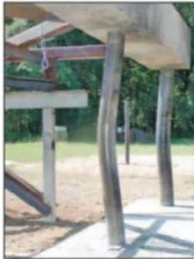
Buckled Steel Column
